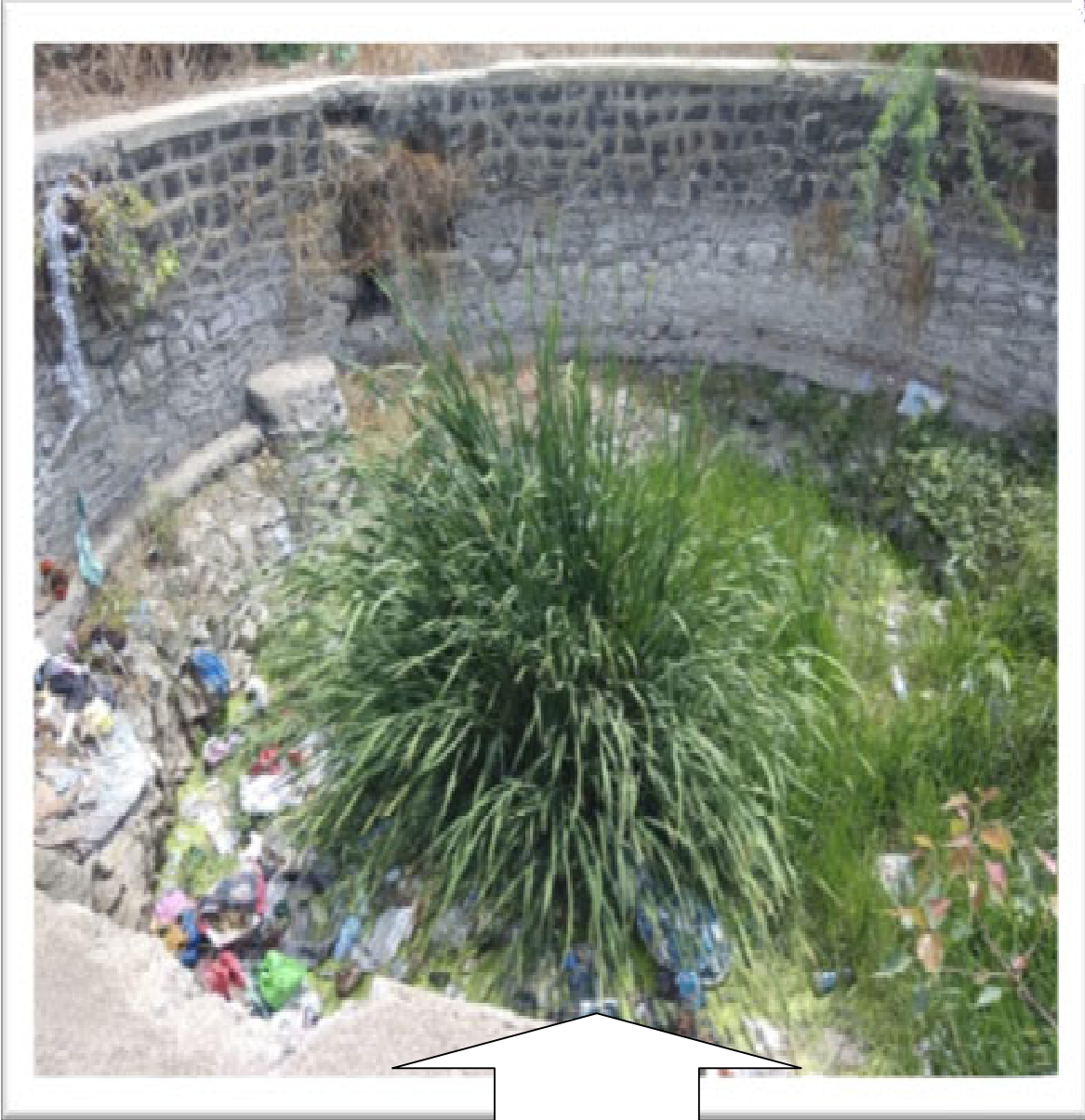
Close view of well located at flowers Quarter, medical college road, this well is filled by wastages, required to Desilt
