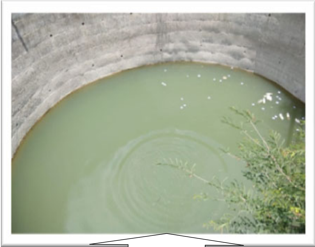
A well located at Company Bag – Depth 30 ft. Water level 12 ft.
