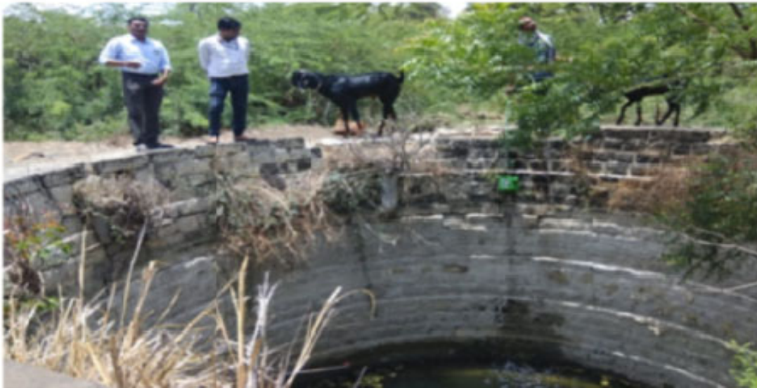
A well located at Company Bag – Depth 30 ft.
